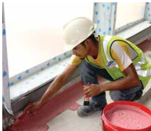
Applying firestopping material at a curtain wall at Tanjong Pagar Centre.
